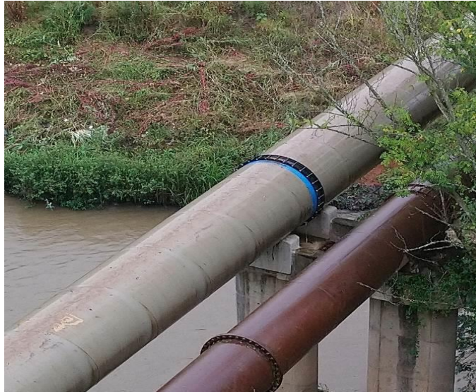
Bridge 2 replaced failed DN1500 with new DN1800
