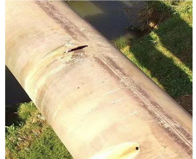
Bridge 1, DN1500 corrosion to crown of pipe replaced with steel patch
