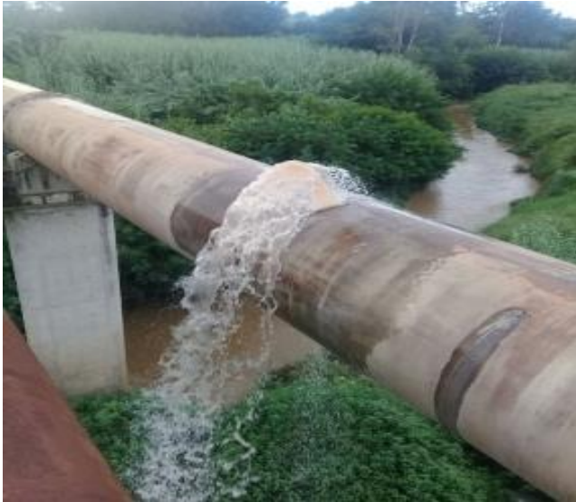
Bridge 1 failure as a result of corroded weld
